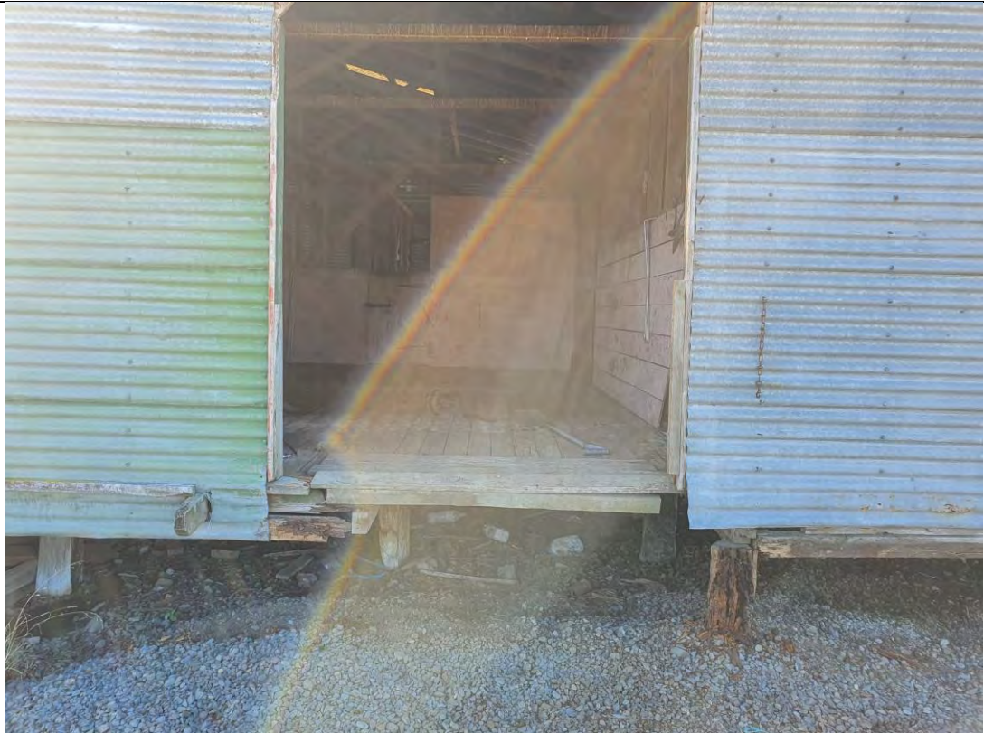
PLATE 7: Western Edge of woolshed showing different ages of corrugated iron and foundations in poor repair
