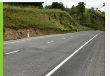
Pōrangahau Road Retaining Wall 184 Downer Complete
