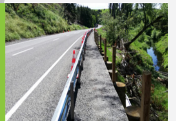
Pōrangahau Road Retaining Wall 434 Downer Complete
