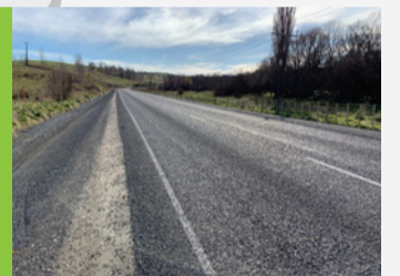
Flaxmill / Wanstead Rooding Upgrade Separable Portion 1 Russell Roads Complete
