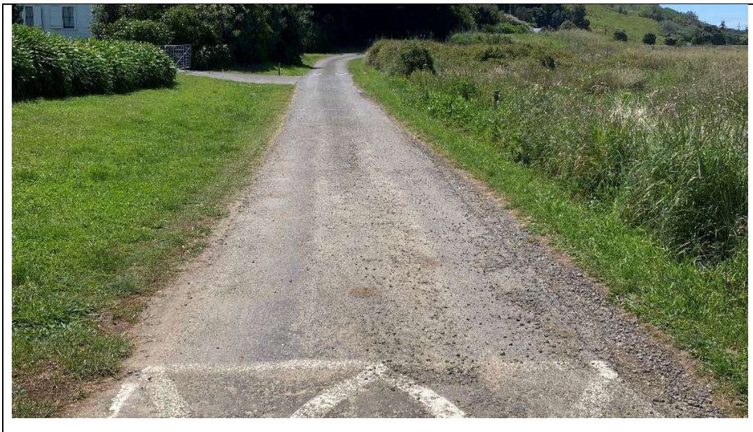
Figure 5 – Okura Road, looking north from site access
