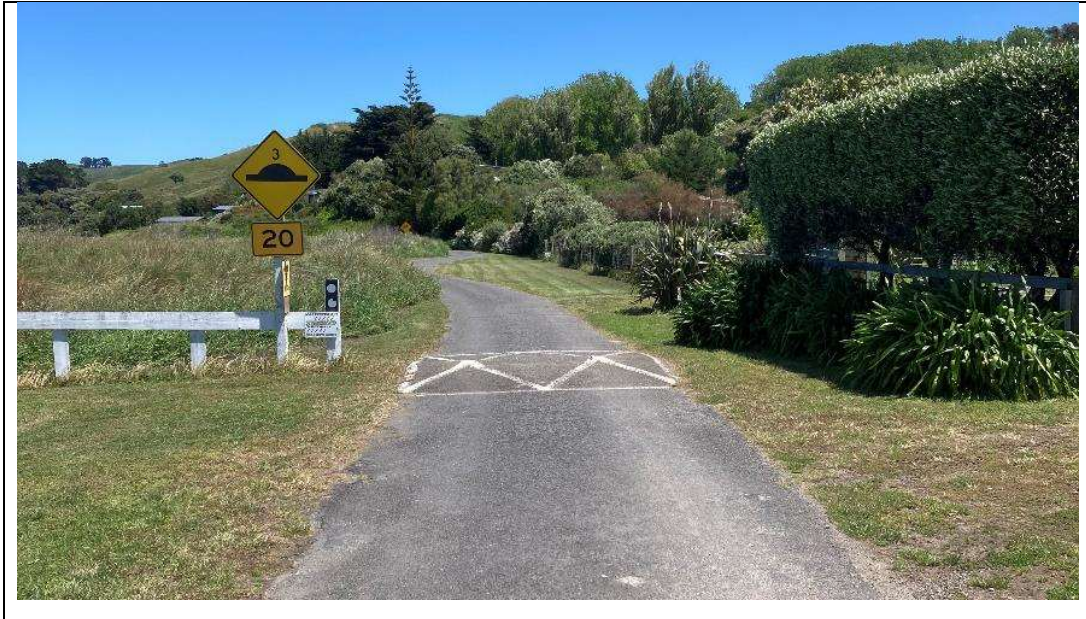
Figure 4 – Okura Road, looking south from Williams Road
