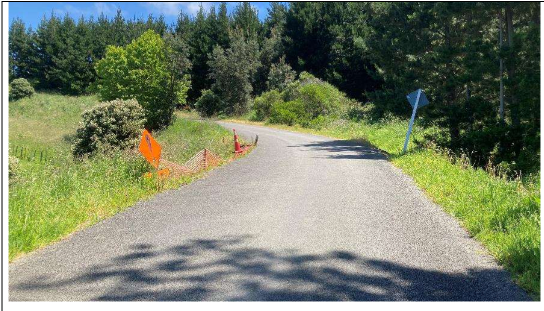
Figure 6 – Williams Road, looking west (leaving beach)
