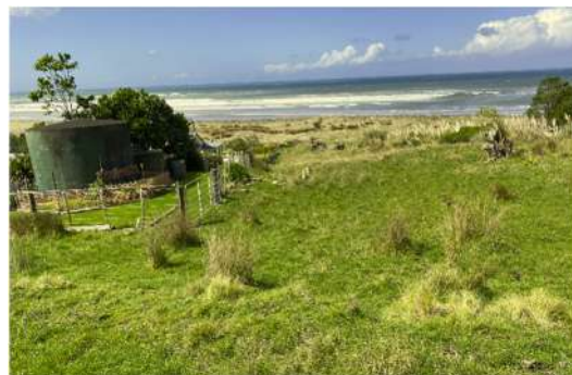
Figure 8 - site photo looking east in approximate location of lot 1-2 access
