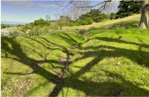
Figure 17 - Existing cut-off drain uphill of 40 Okura Road
