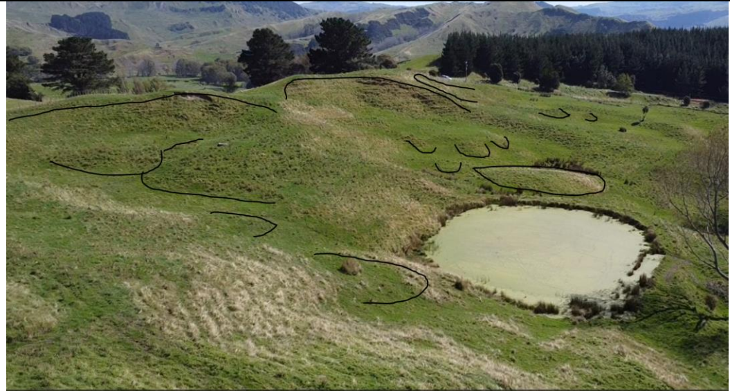
Example of Seismically induced Landslide and debris flow below Lot 7 (left) and Lot 6 (central).
